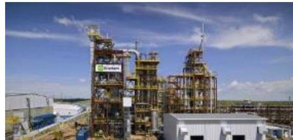
EDMONTON – 1 ST FULL SCALE FACILITY
